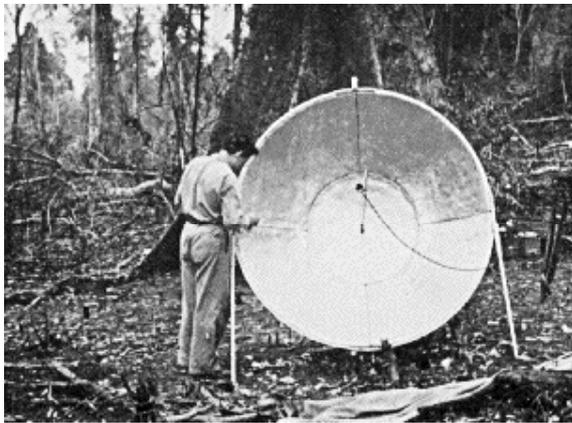
Clarence R. Carpenter at Doi Dao (north of Chiangmai, Thailand) in 1937, with the parabolic reflector which was used for making the first sound-recordings of wild gibbons (from Carpenter, 1940, p. 26).
